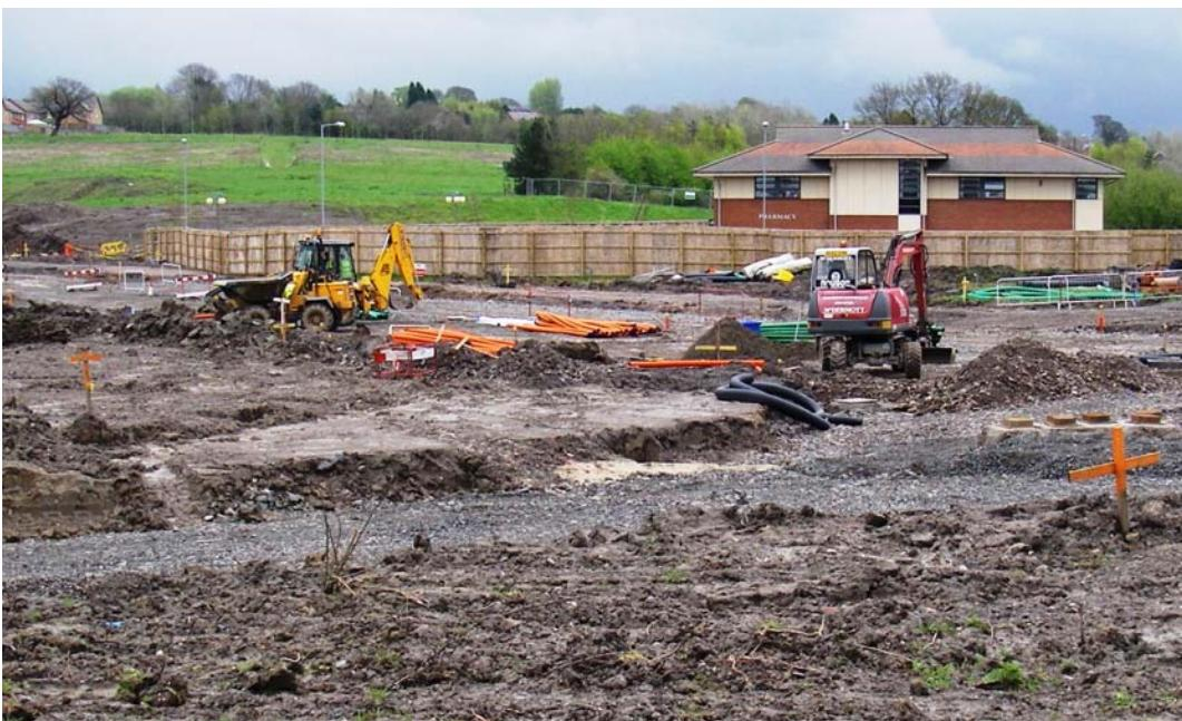
GeoDyne obtained sufficient information to recommend various foundation options on variable engineered fill materials up to depths in excess of 8m. Localised anomalies (i.e. buried highwalls associated with former coal opencast workings) were also identified in sufficient time to allow our Client to take into consideration potential abnormal development costs.
