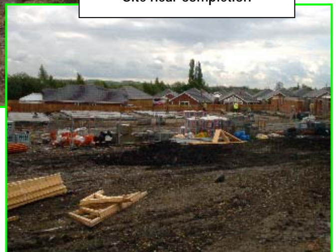
Site near completion
