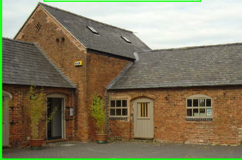
GeoDyne Office in Radbourne
