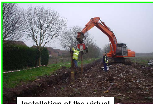
Installation of the virtual curtain nodes
