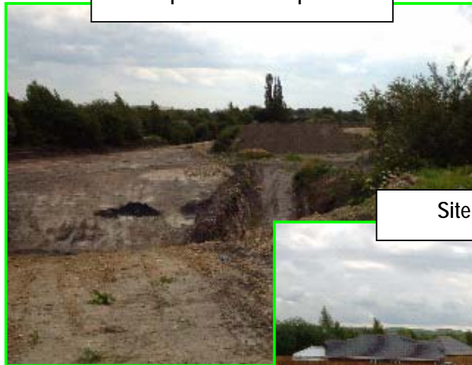
Site prior to development
